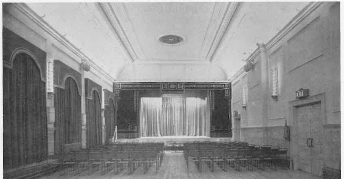
Translucent cornice lighting with fluorescent lamps in the Town Hall, Maidenhead.
