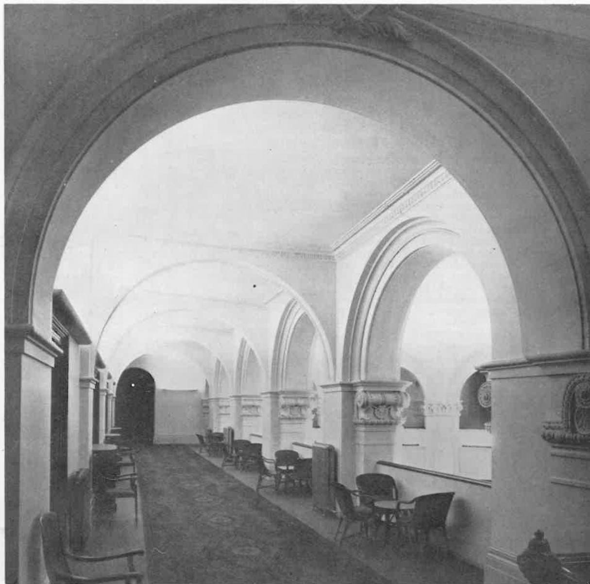
Indirect fluorescent cornice lighting in Grand Hotel, Scarborough.
