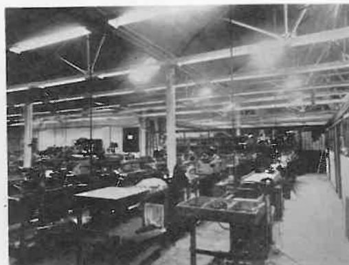
2 Another early Mazda fitting, with lamp control gear held in chain suspension, was installed during the war in underground caves at Corsham where a vast aircraft factory was located.
