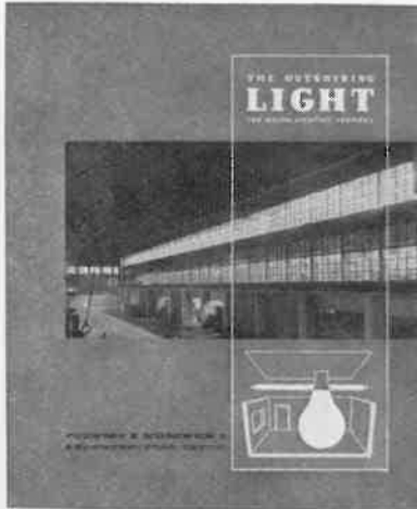
Cover picture shows a night view of the Vauxhall factory at Luton. Lines of fluorescent lighting, photographed in a disappearing perspective, guide the eye along the whole length of the highly glazed exterior.
